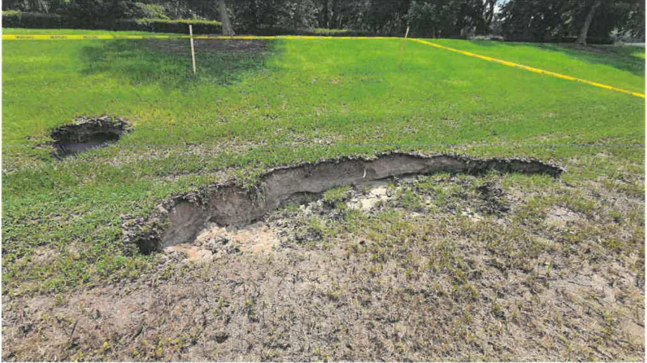
Site Photo No. 1 – Surface Depressions in DRA 8 located at Indigo East South in Ocala, Florida
